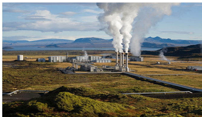
Geothermal Power Production in Naivasha , clean and affordable energy for growth.
