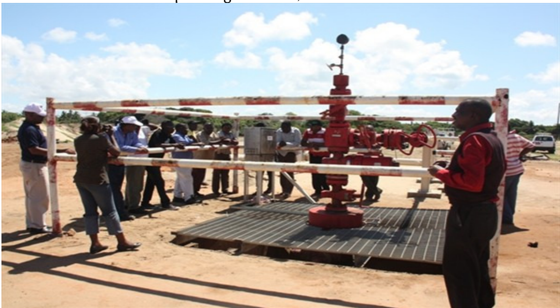
The photo shows one of the Natural Gas Well at Mnazi Bay - Mtwara
